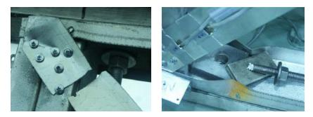
Figure 7. Potential undesirable failure modes in flat strap shear walls (corresponding to DS3): (a) Improperly detailed connection leading to net section failure; (b) Improperly sized rod leading to anchorage failure (image source: [20])
